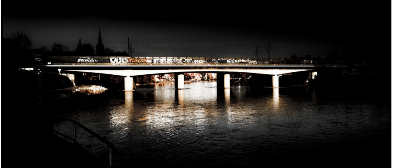
Train Bridge I
